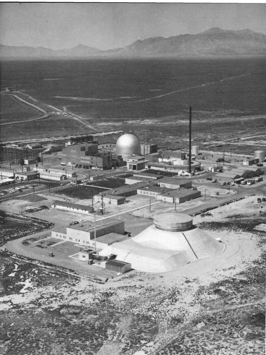
Figure 11 Exterior view of EBR-II buildings. The reactor is housed in the dome-shaped structure.
