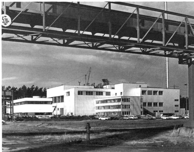
Figure 19 West Germany's KNK experimental nuclear power plant.
