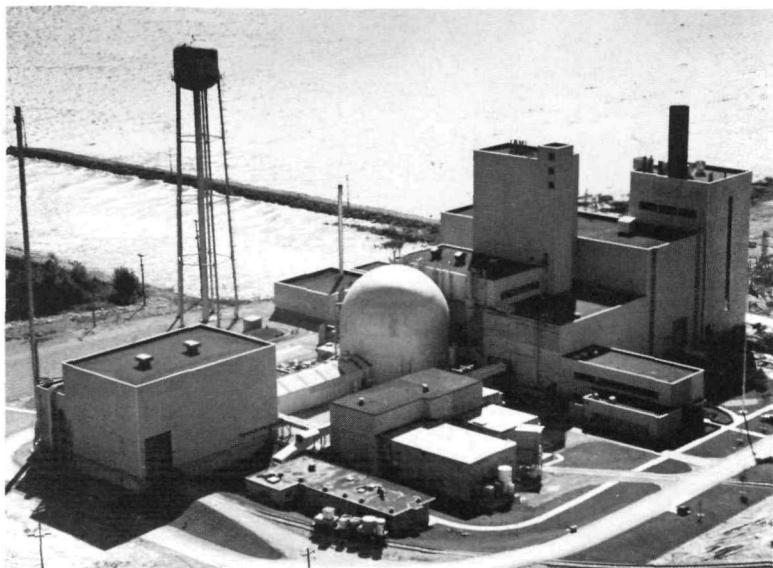
Figure 12 An aerial view of the Enrico Fermi Atomic Power Plant.
